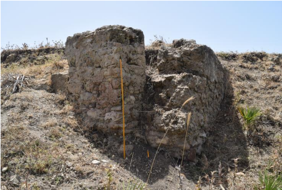
Figure 8. Standing architecture of a thermal complex (TU0076), so-called "Graza." Taken from the bed of the Oued Rayhane (Photo: S.C.-E.).
