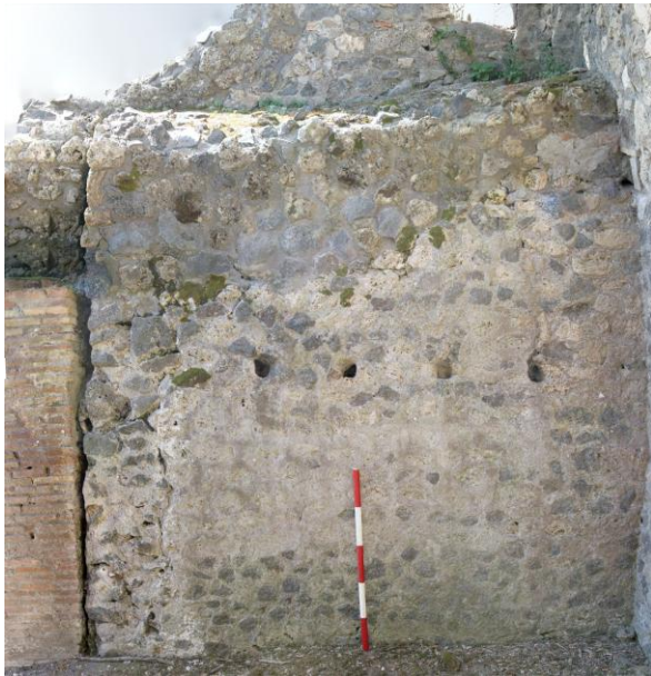
Fig. 9. Wall face 265 (room 37), from North.
