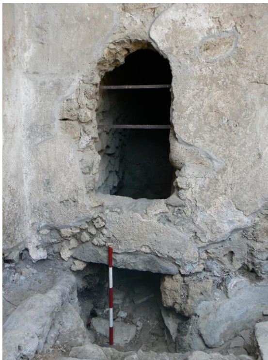
Fig. 13. Original sewer line and cut through its floor. Curve of the new sewer and the cruma bedrock are also visible in the cut.
