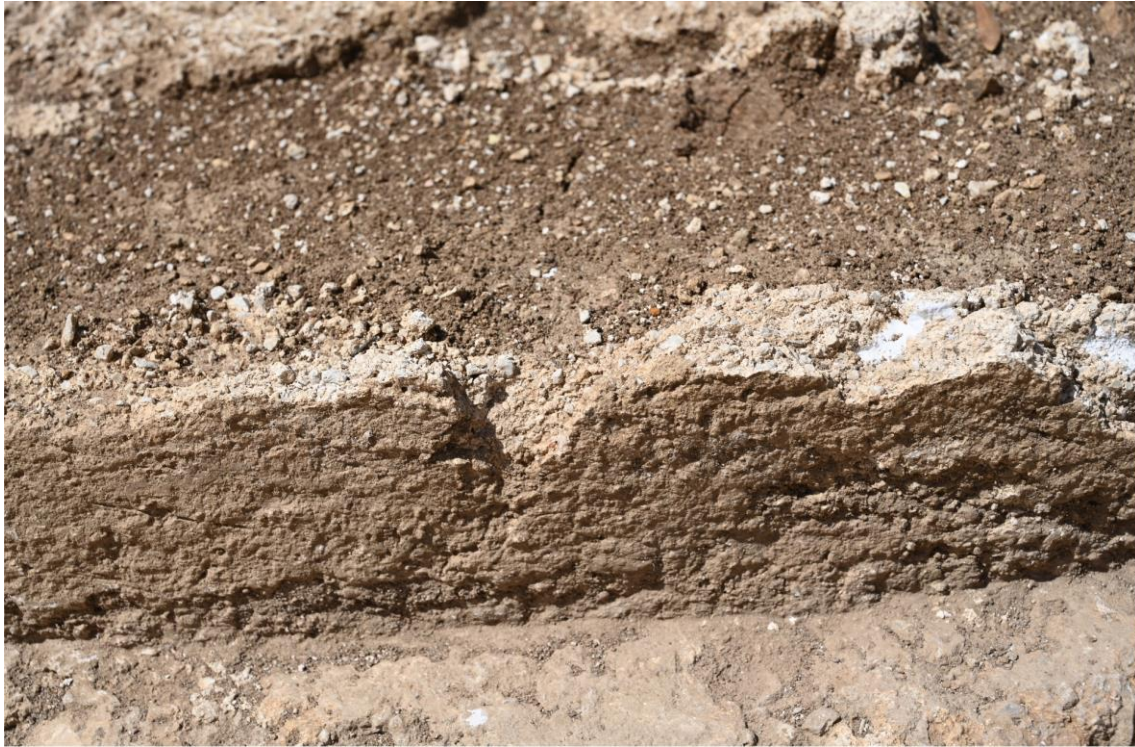
Fig. 9. Detail of the fill within the cob, pise or opus craticium walls and the wall's exterior surface, Room 8a. Martin Beckmann, McMaster University.
