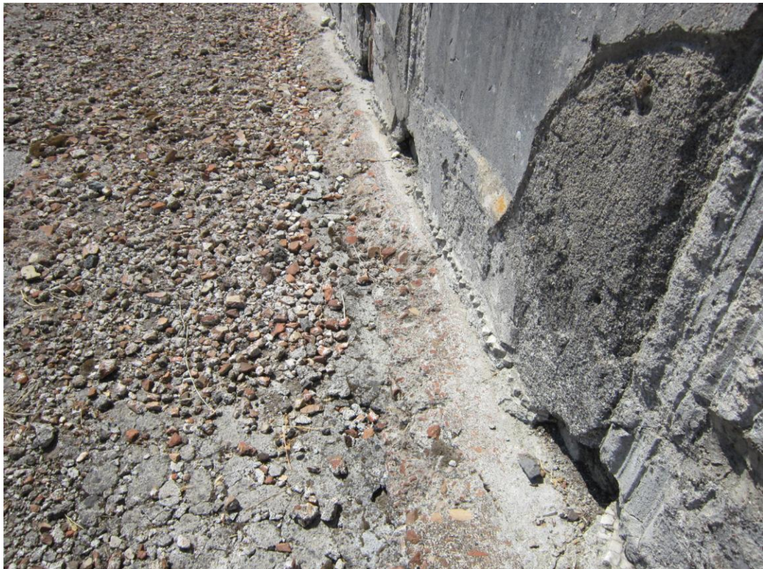
Fig. 6. Temple of Apollo, detail of podium and east flank of cella showing white tesserae bedded on a cocciopesto pavement and pinned under stucco wall decoration; from the northeast.
