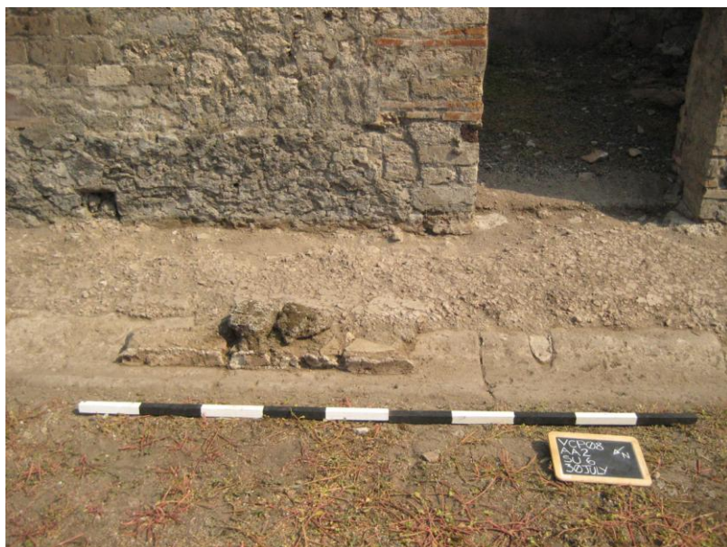
Fig. 32. Low dividing wall built directly over tufo nocerino channel.
