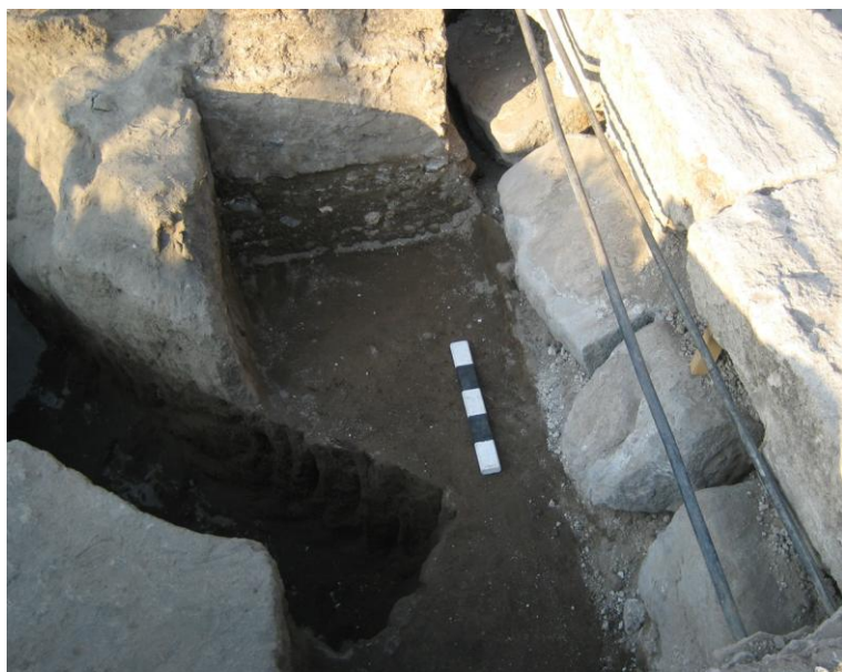
Fig. 28. Collapsed kerbing stones on southern side of AA001.
