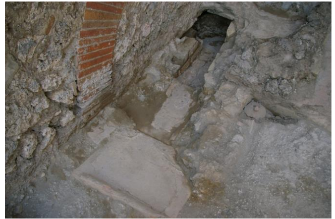
Fig. 7. Taberna V 1, 2: drainage installation.
