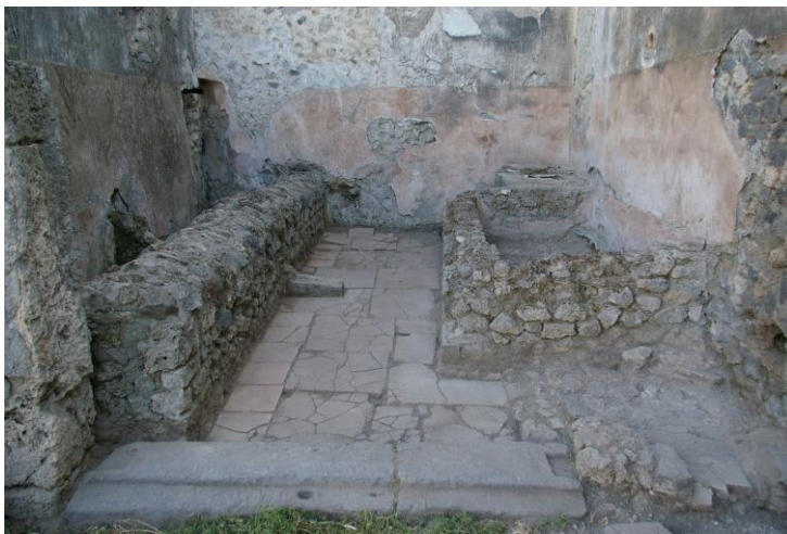
Fig. 15. Workshop VI 16, 3.4: room I, overview.
