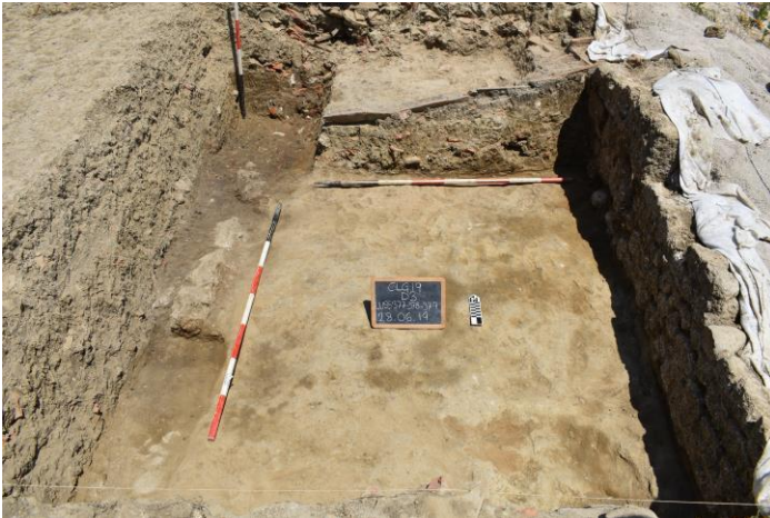
Fig. 23. Excavation area D3 (2019); view north. Segment of early stone wall is visible to the west; the back wall of the bath complex is to the east; and late pan tile drain is to the north (photo R. Schindler).
