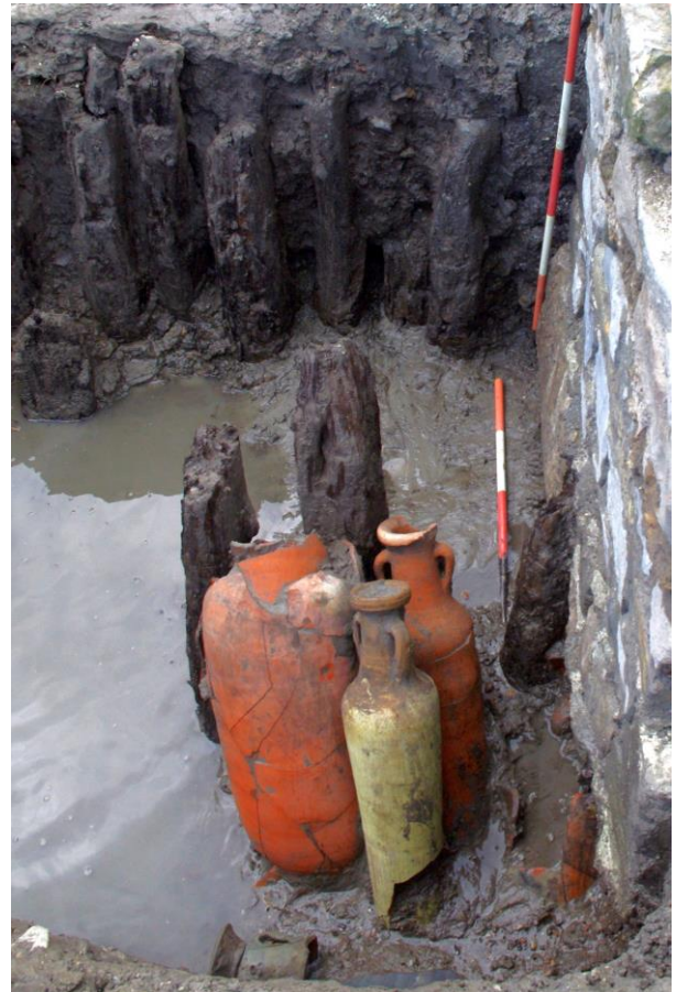
Fig. 6. Site 1. The timber piling and land consolidation amphorae put in place prior to the construction of the outer curtain wall (photograph Patrizia Basso).
