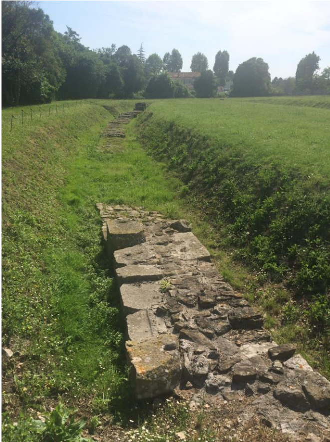
Fig. 5. The outer curtain wall (photograph Patrizia Basso).
