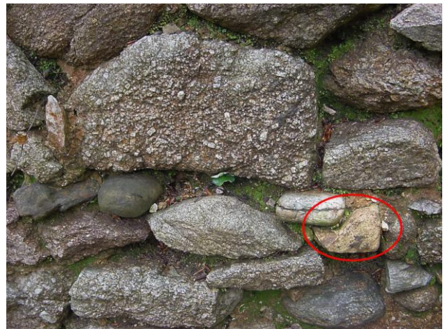
Fig. 3. Contrada Palazzo 2014. Detail of the western wall (seen from the southwest) with Greek pantile fragment embedded in the masonry.
