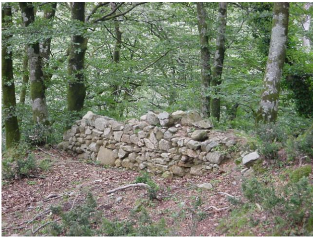
Fig. 2. Contrada Palazzo seen from the southwest in 2013. Remains of the western wall with large granitic block in the bottom course.
