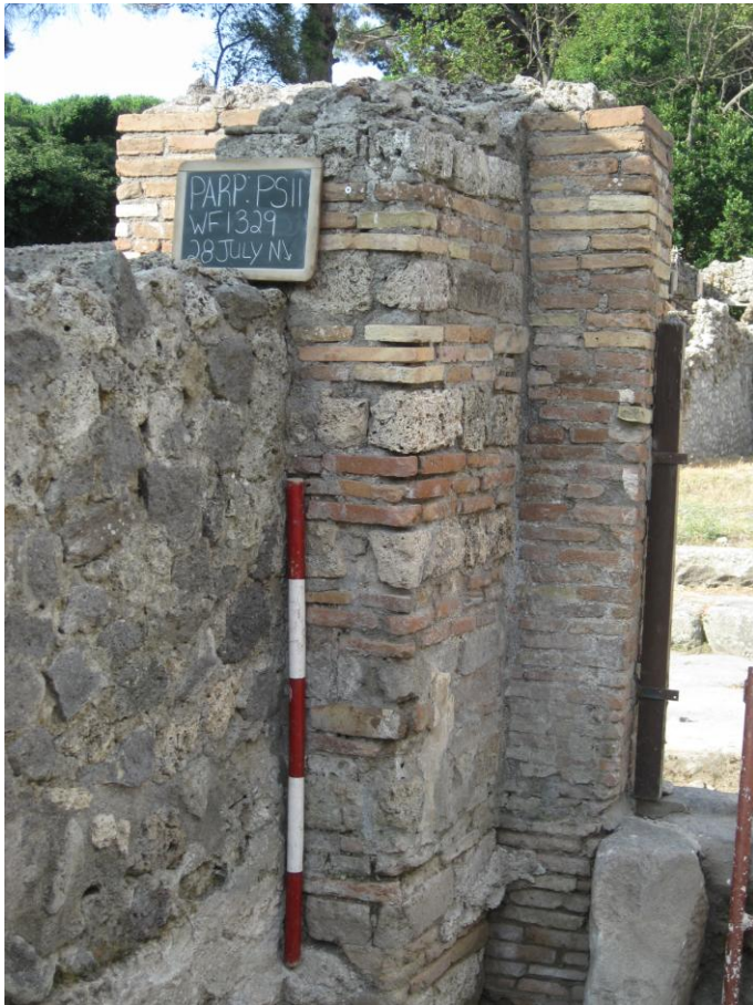
Fig. 26. Quoin of opus mixtum, looking west. Note the later additions of the brick quoin to the right and the opus incertum wall at left (Phase 11).
