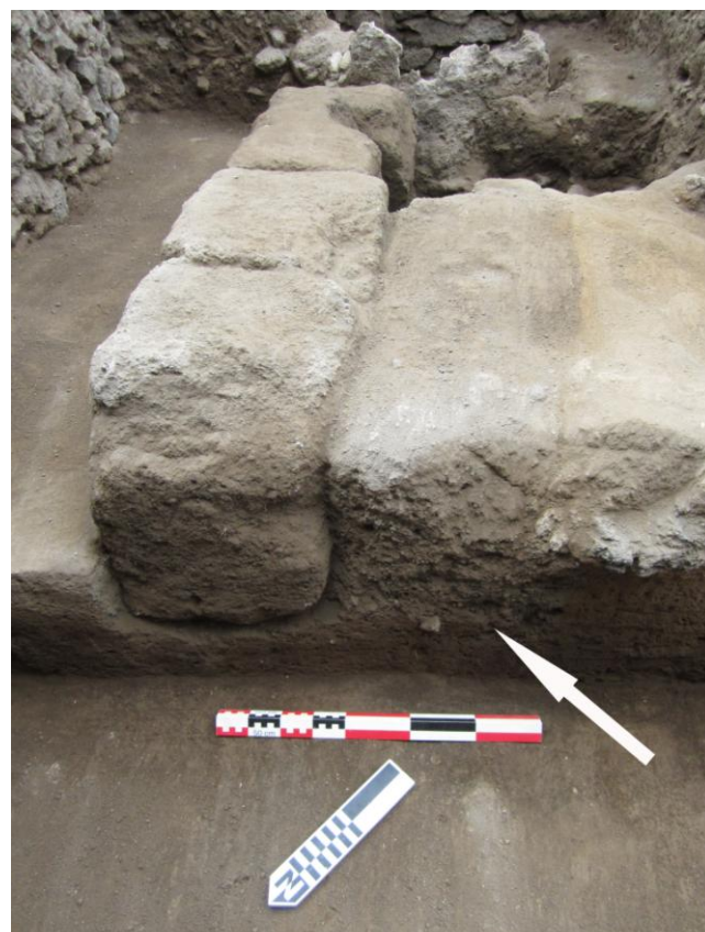
Fig. 14. Detail, in cross-section, of the construction trench for the pappamonte wall and its construction fill (at right).
