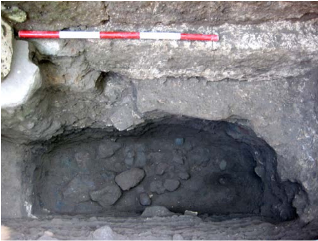
Fig. 32. The first foundation layer for the construction of the Porta Stabia.
