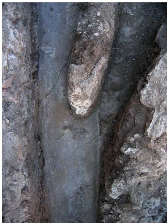
Fig. 18. Detail of the later attachment of the second drain, at right.
