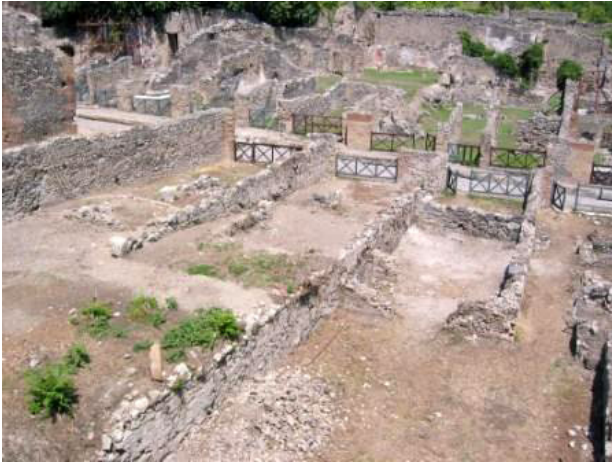
Fig. 31. The eastward continuation of the terrace wall. Note the difference in elevation from one side to the other.
