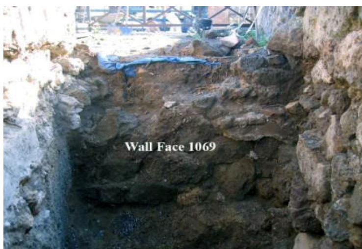
Fig. 18. Wall Face 1069 projecting north from the division wall, at right (Wall Face 235).
