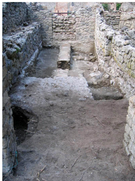
Fig. 9. Note the blocking of the doorway at the eastern end of the room (from Phase 4).
