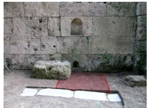
Fig. 34. The two arched shrines cut into the east wall of the Porta Stabia. Location of Trench 10000 indicated by red shading.
