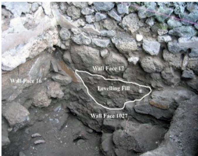
Fig. 14. Early wall (Wall Face 1027) on a north-south alignment. Note its destruction and subsequent levelling fill for the following sequence of construction.
