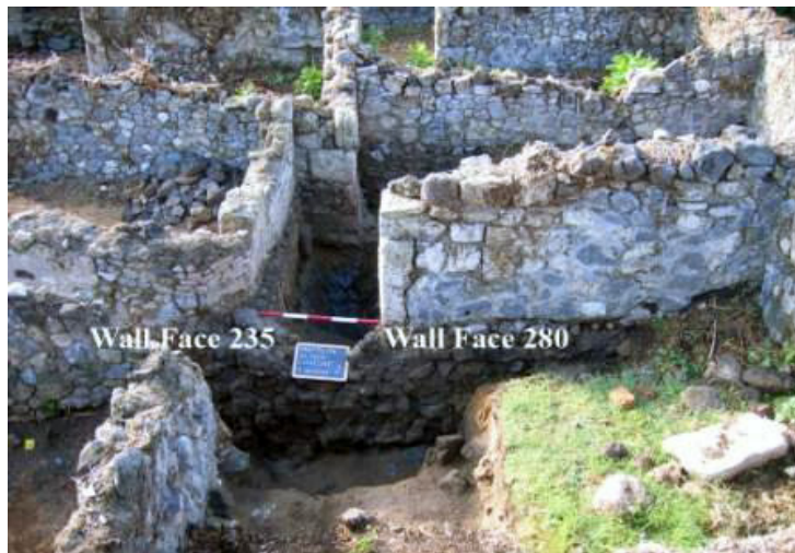
Fig. 17. The unified construction of Wall Faces 235 and 280. The doorway was created in the fourth phase.
