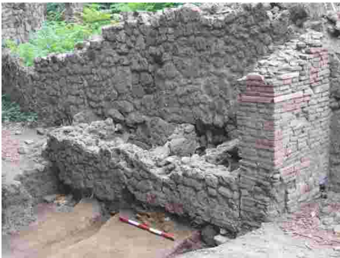
Fig. 19. The industrial tanks
