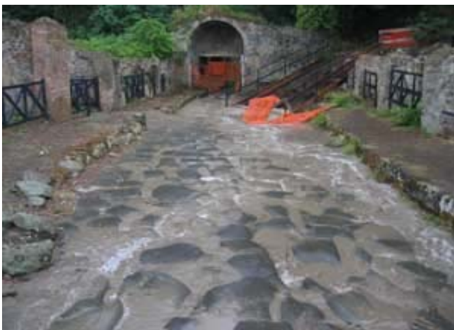
Fig. 28. The rainstorm, with water directed toward the drain
