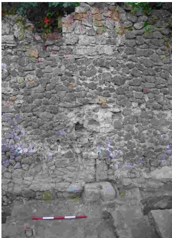
Fig. 18. The southern property wall
