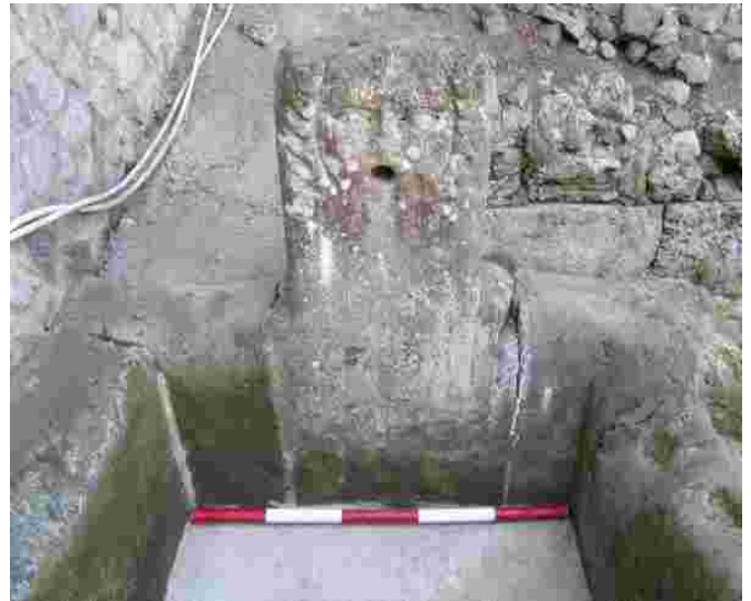
Fig. 27. Detail photo of wear on the rear wall of the fountain
